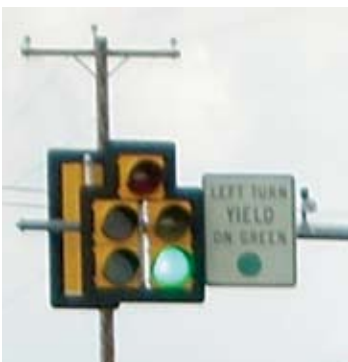
Typical Protected-Permissive left turn signal head
