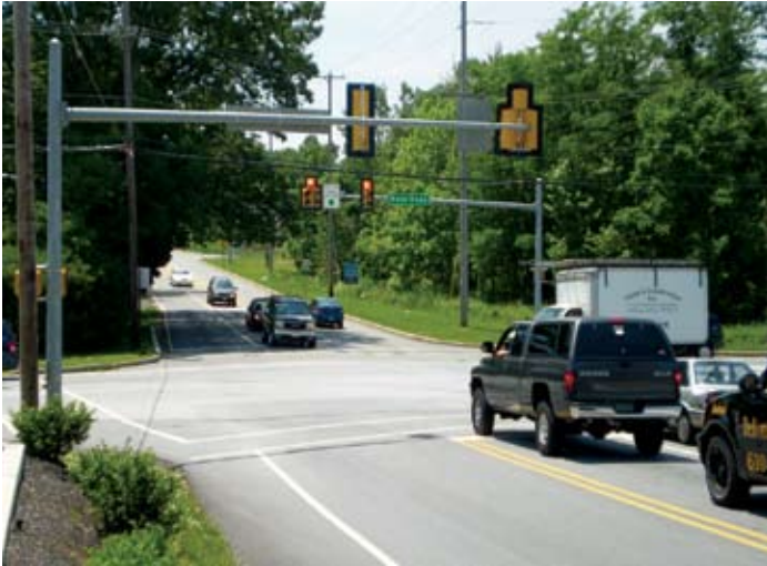
An intersection similar to this one, fully actuated with a high volume of left turns will benefit from cross switching.
