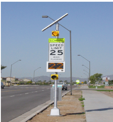
Figure 3 - Speed display with LED school beacon system, Goodyear, AZ
