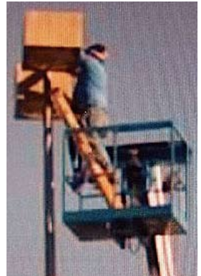
Above: The worker is 40 feet in the air working on a parking lot light in a JLG lift . . . Notice the ladder in the cage area and he's not wearing a harness.
