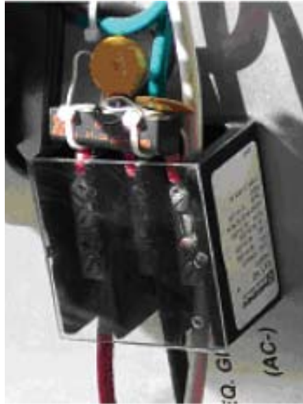
Gas-tube and MOV AC protection – grossly inadequate
