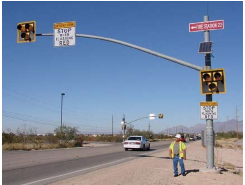
Figure 5, City of Tucson fire station exit signal with "Mickey Mouse" signal head
