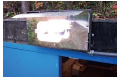
IL with cover removed. The lamp is large and precise distribution is difficult to obtain.
